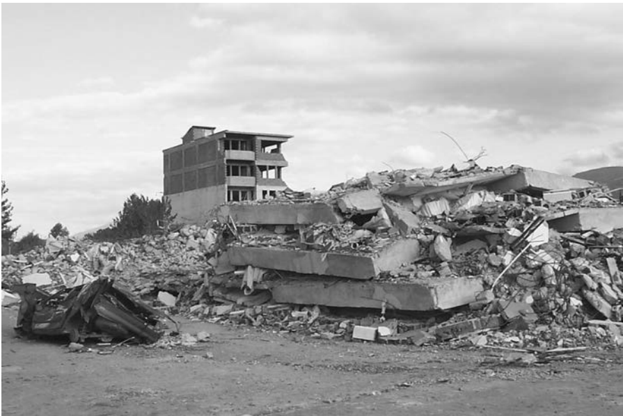
Fig. 4.4 'Pancaking' of Multistoried Structure in Area of Cyclic Mobility, Turkey. Photo: R. Rothaus.
